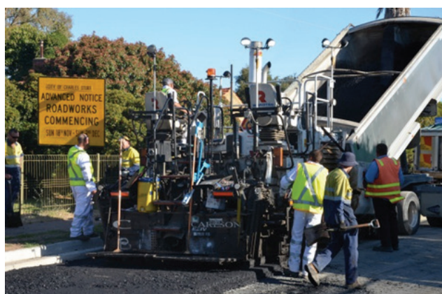
Laying of new asphalt surface
