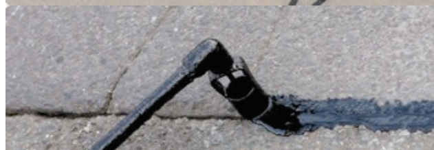
Crack sealing
