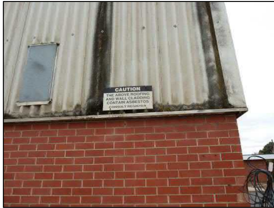
Photograph 27 – View of asbestos containing material Building 404 in the north east of the site
