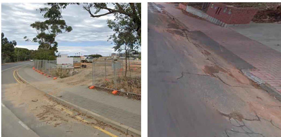
Figure 7.13 Examples of development sites, with visible sediment at the entrance to the site and on the downstream road network.
