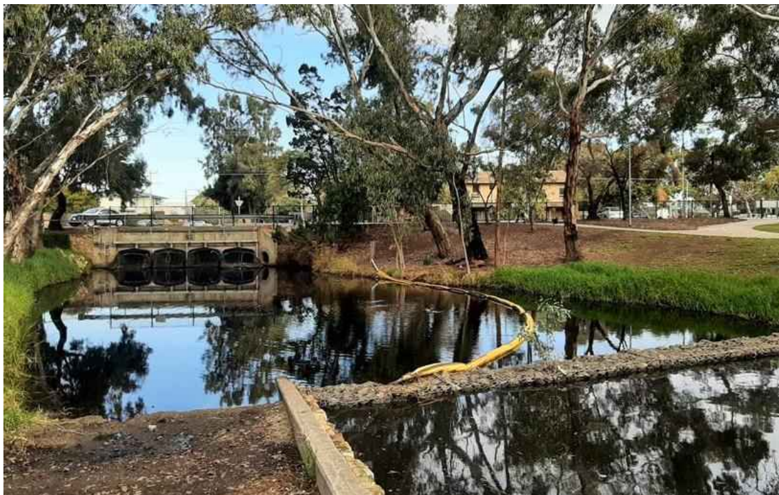
Figure 7.11 Trash nets at the upstream end of the Grange Lakes channel
