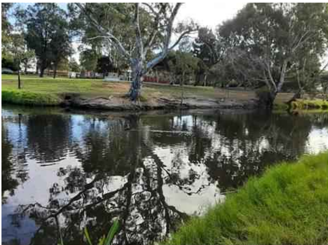
Figure 7.9 The Grange Lakes natural section of channel – note the exotic grasses and erosion on the bank, with steep drop off into the water.
