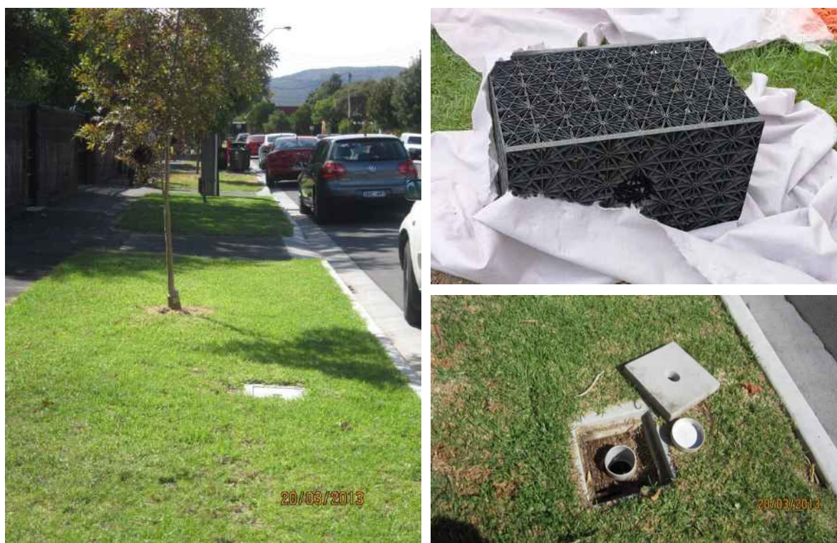
Figure 7.3 Burnside Council's B-Pods (watersensitivesa.com)
