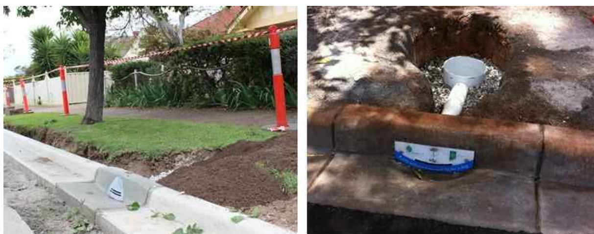
Figure 7.4 TREENET Pit inlet and infiltration pit (City of Mitcham, watersensitivesa.com) and City of Holdfast Bay (https://www.yourholdfast.com/wsud)
