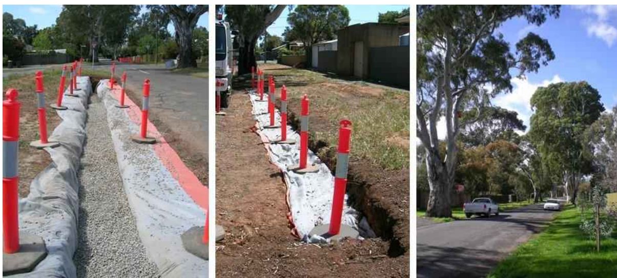
Figure 7.5 Infiltration trench, supporting roadside vegetation in Colonel Light Gardens (watersensitivesa.com)
