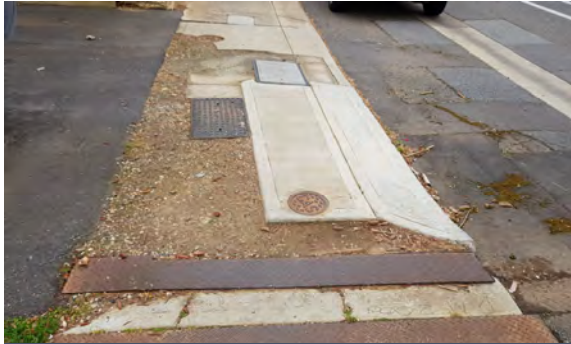
Cracked/uneven footpath pavement
