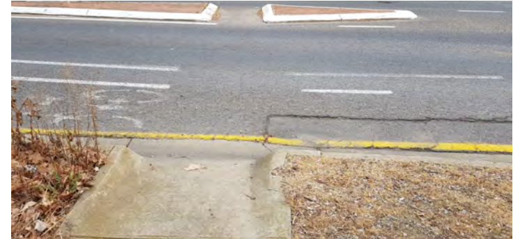
Non-compliant kerb ramps/crossings
