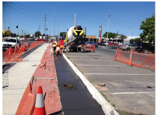
Laying of New Path Surface
